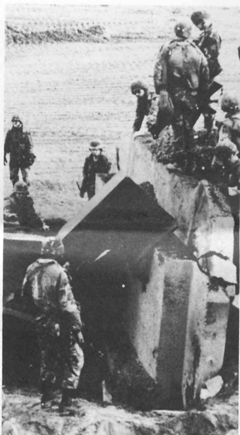
And aftermath ... The same S-bahn bridge after the engineers demolished it.
