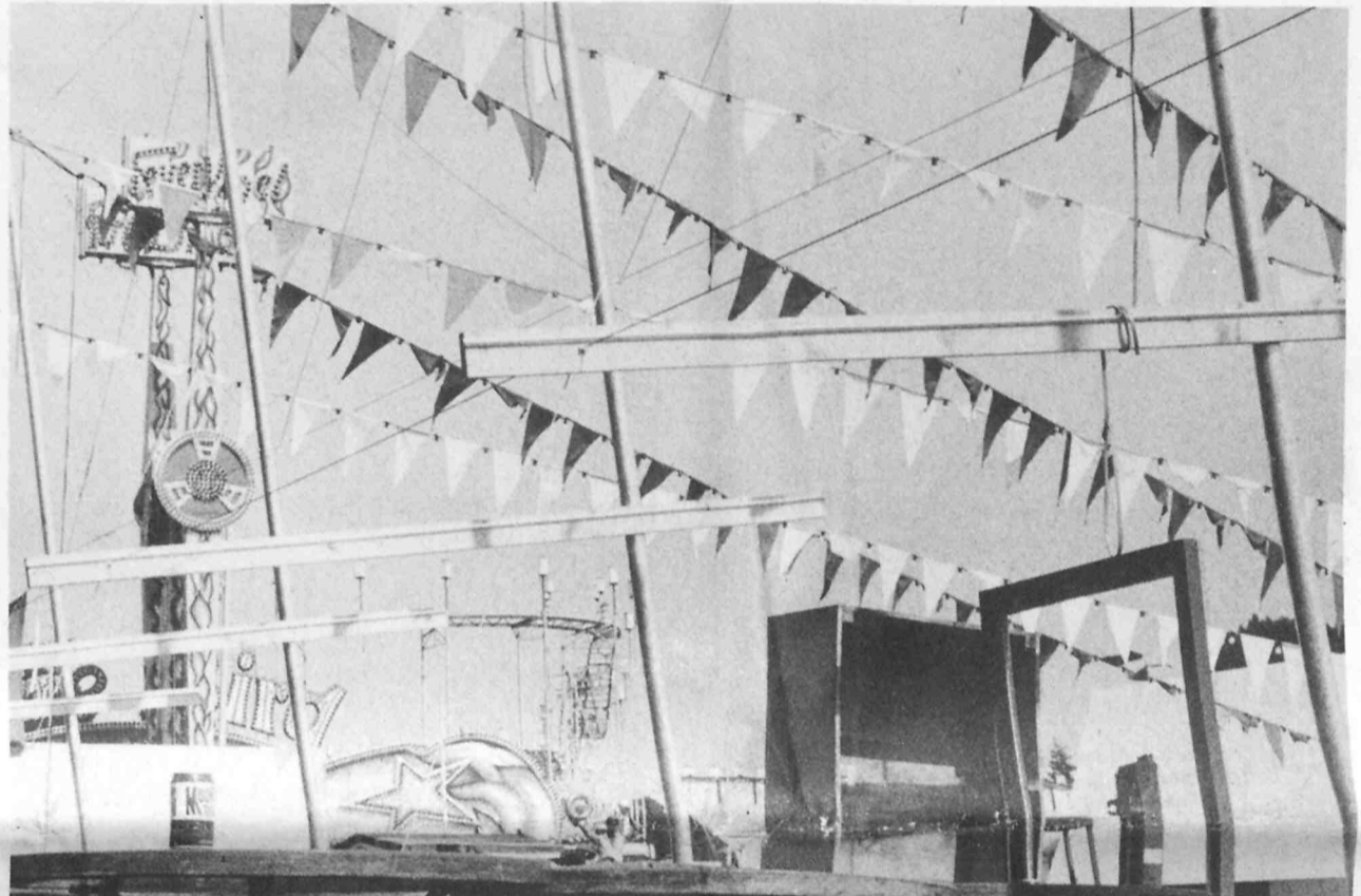
Taking shape . . . The skeleton of Volksfest rises from the YA parking lot.
