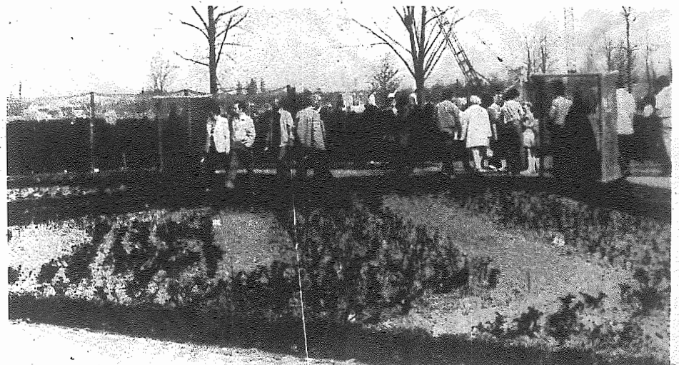
Strolling through the almost completed rose gardens
