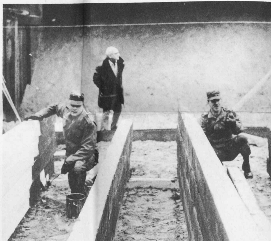
BAFFLES?—Sp4 David Weedall and Pvt. Dalton Withby put preservative on the 6x8 wooden beams that will be
