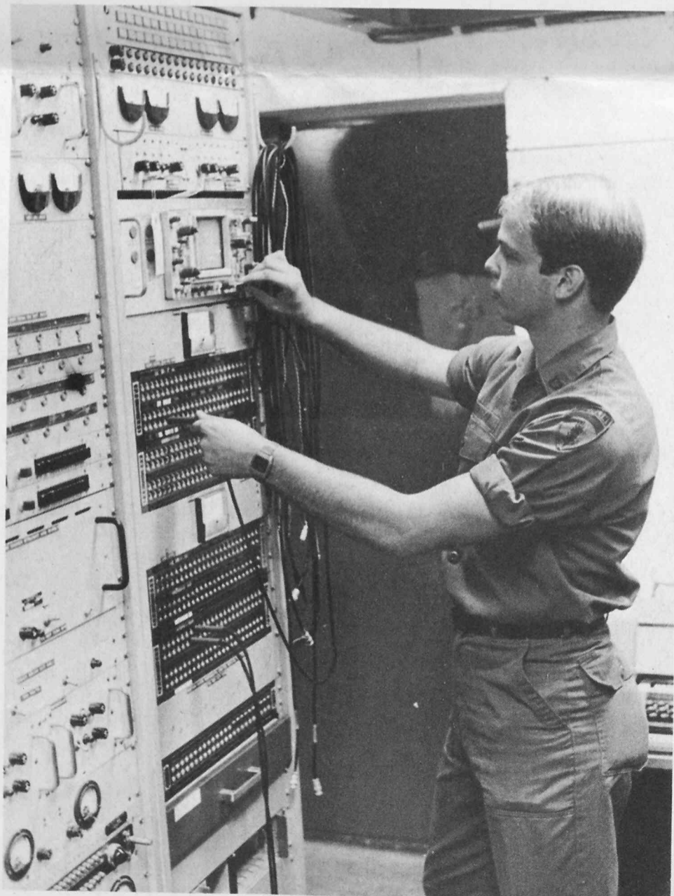
SCOPE-ING IT OUT—PFC Vincent R. Conrad uses an oscilloscope to check phone line inputs in the
