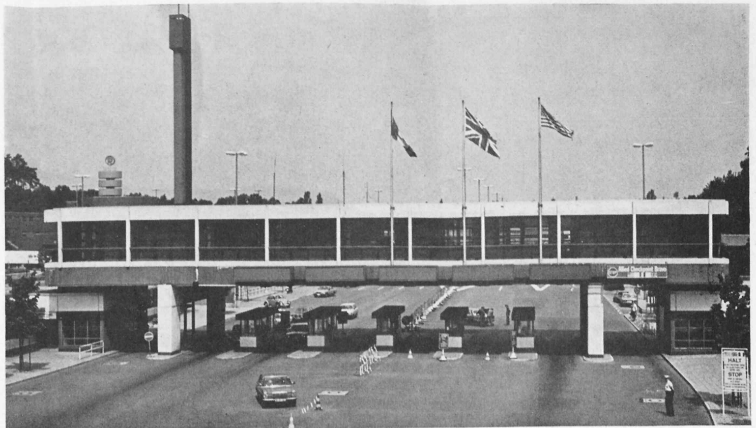
WELCOME HOME — Travelers driving from Berlin to Helmstedt on the autobahn must process through Allied Checkpoint "Bravo." At the checkpoint, travelers receive a safety
