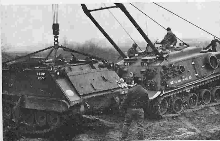
THE CRIPPLED APC BEING LIFTED BY THE VTR.
