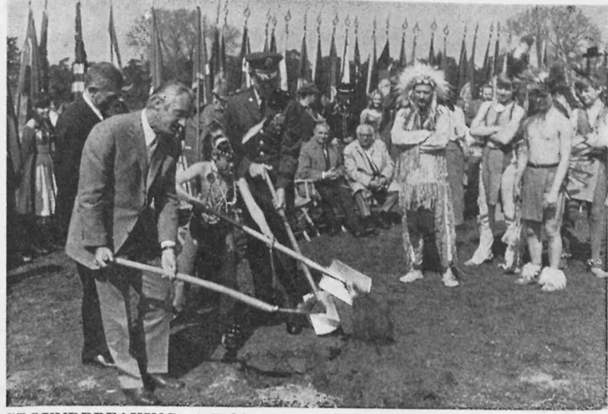
GROUNDBREAKING — Taking the first shovels full of dirt, marking the start of preparations for the 1971 German-American Volksfest, "The Wild West" are, from l. to r., Zehlendorf District Mayor Hans-Joachim Schnitzer, Thomas Sharper, Brigadier General Harold I. Hayward, commanding general, Berlin Brigade, and the "Indians." Looking on behind Mayor Schnitzer is David L. Klein, American Minister in Berlin, who participated in the earth turning and then relinquished his shovel to young Sharper.
