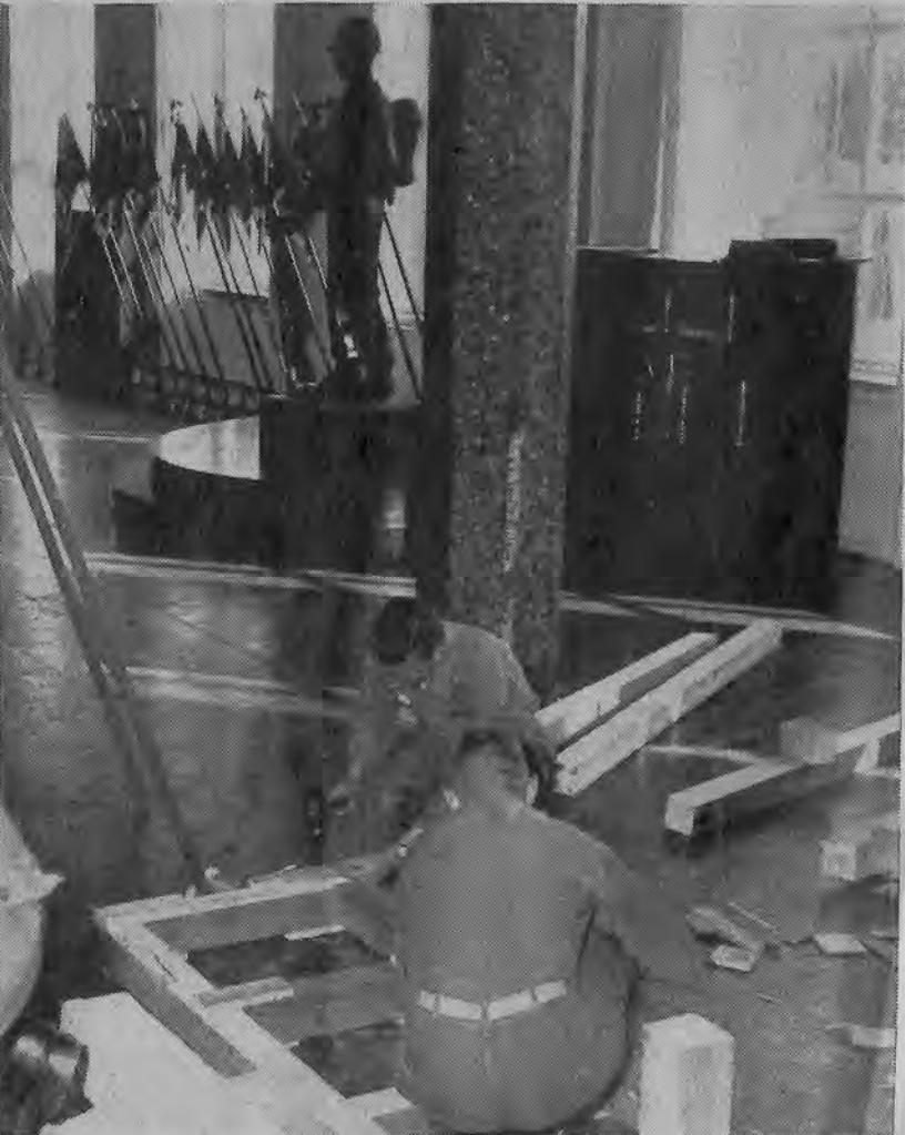
Present construction projects are "changing the face" of McNair Barracks ... here, the 2nd and 3rd Battle Groups' Hall of Honor begins to take shape ...
